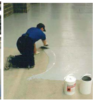
Trowel application ensures an even distribution and consistent finish
