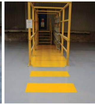
Professionally installed floor markings give clear health and safety information
